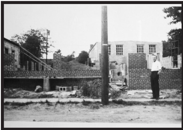
Stephan J. Schaffan Sr. oversees the construction of the first Atlas track factory in Hillside NJ.
